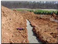
Begin by digging a two foot wide trench. Excavate all loose soils and native rock until hard original ground is reached. The footing will be supporting the entire weight of the wall.
