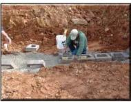
When laying the first course, level the block front to back and side to side with a two foot carpenter's level. It is very important that the first course be placed on a compacted footing and leveled before preceding.
