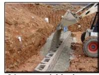
It is recommended that the cores of the block be filled with a #67 or #78 stone no less frequently than every three courses. This same stone is recommended for the backfill as well.
